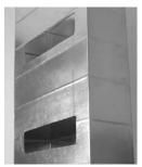
Tape template to return air plenum. Cut opening with metal shears, predrill for the securing screws and remove template.
